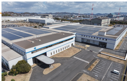
Sumitomo Heavy Industries Gearbox Co., Ltd. Okayama Factory (Okayama, Japan)
